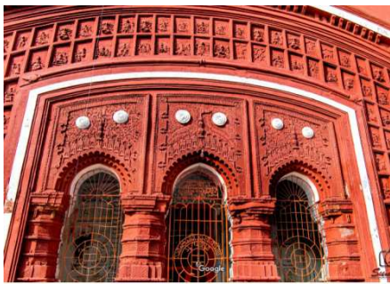
The terracotta panels in the facade
