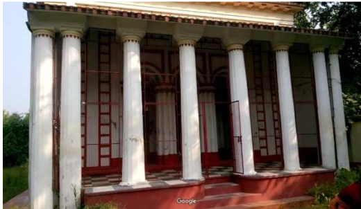
The doric columns at the porch.
