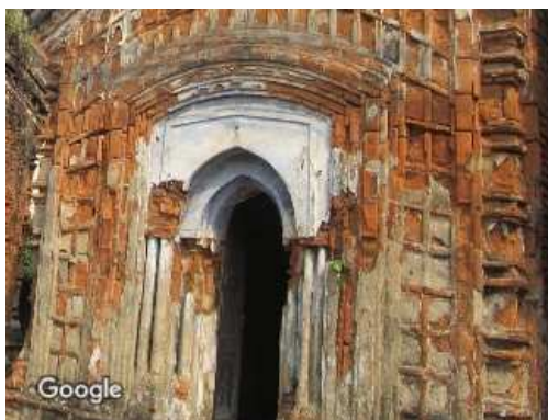
The arched entrance and the coffered terracotta walls
