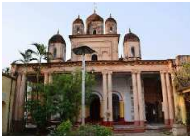
Good/Fair/Showing Signs of Deterioration Advanced State of Decay/Danger of Disappearance
