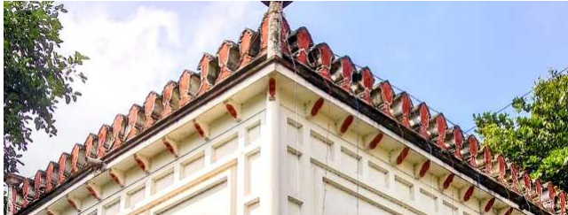
The cornice and the decorative parapet
